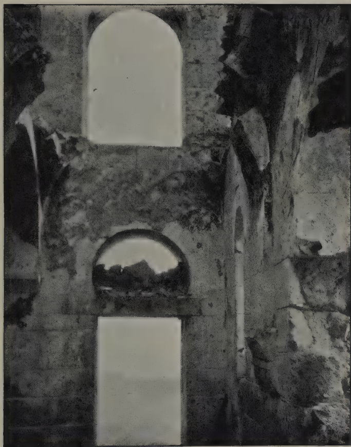
FIG. 336.—Tchangli Klisse, interior of narthex, looking S.
